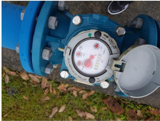
Figure 2: Bulk meter capsule reading
