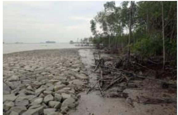
Rock revetments along the coastline of Tanjung Piai to protect against accelerated erosion.
